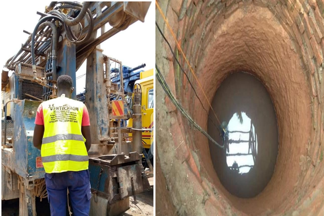
Water sourcing and rehabilitation works
